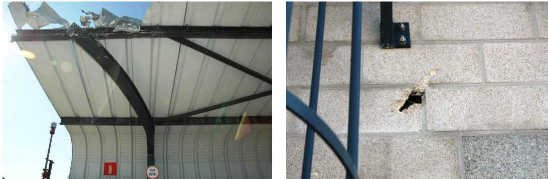
Figure 4: Pictures of the roof's damage and damage to the concrete wall of the tower.
